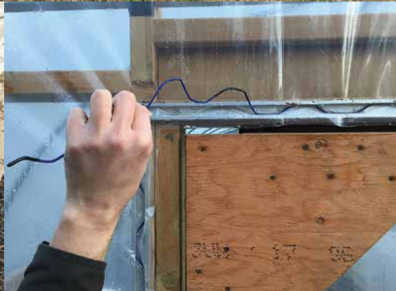
Wiggle wire secures the tunnel's plastic coating to the frame in a wire lock channel (also called a poly latch). The same wire can be re-used when it's time to replace the plastic.
