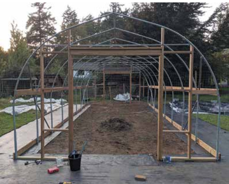
The completed frame and walls of the high tunnel. The gothic-style peak of the roof is visible, designed to avoid the accumulation of wet, heavy snow. Photo: Matt Gubernat.
