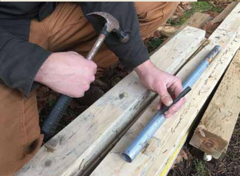
Drilling into the rounded, metal surface of the high tunnel pipe is challenging, so Matt uses a punch to create a registration mark before drilling each hole.
