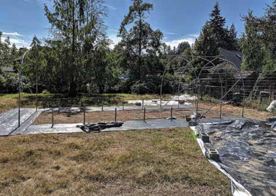
The ground posts of the high tunnel are complete, and Matt has begun erecting the arches. Black landscape fabric surrounds the structure to suppress weeds. Photo: Matt Gubernat.
